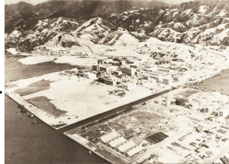
Kwun Tong industrial district (1962), reclamation & factory construction simultaneously (Source: Challenges for an Evolving City)
