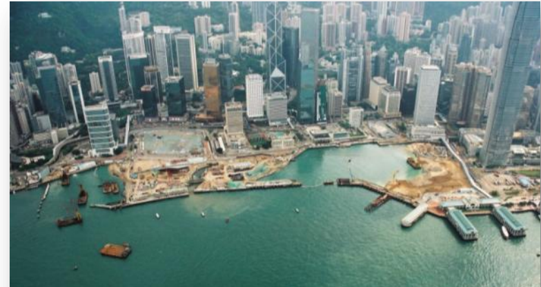
Central Reclamation Phase 3
