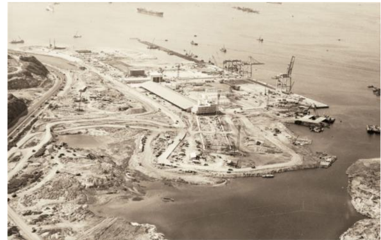
Kwai Chung Container Terminal under construction (1972) (Source: Challenges for an Evolving City)
